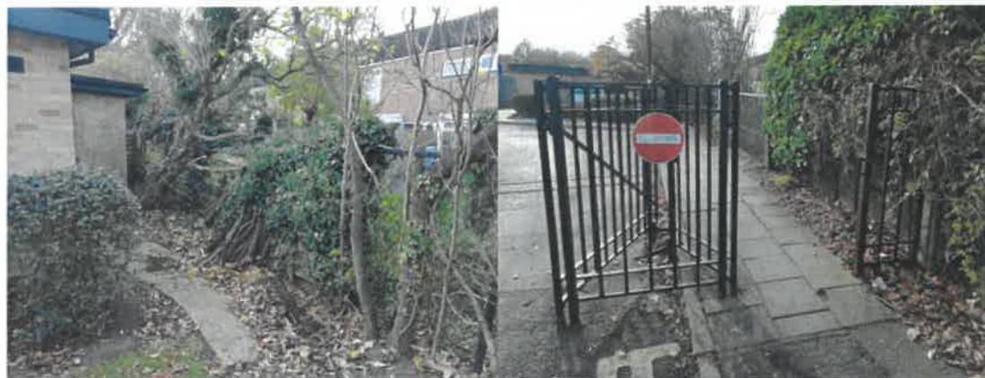
Figure 2: Existing fencing and gate system provision very little protection
