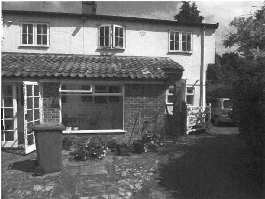
North Entrance, Saxmundham
