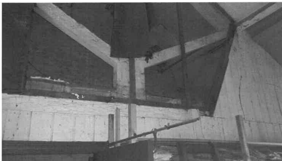
Existing open mezzanine over existing office, wc and stairs
