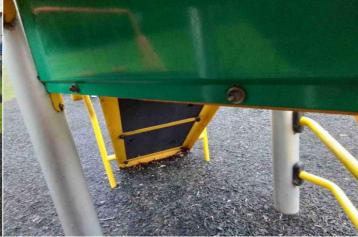
Action: Remove excess thread length and deburr or provide
