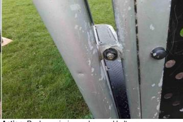
Finding: There is/are bolt cap covers missing or damaged Action: Replace missing or damaged bolt cap covers on the item
