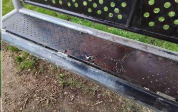
**Finding:** The paintwork on this item has been damaged or worn exposing the metal underneath which is rusting / corroding
