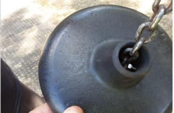
**Finding:** The chain links are worn in excess of 40% and require renewing
