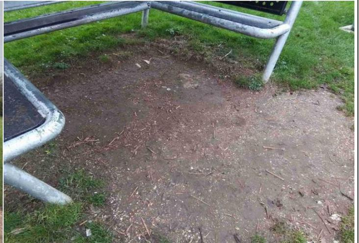
**Finding:** The surface has eroded in some areas and may be slippery in wet conditions
