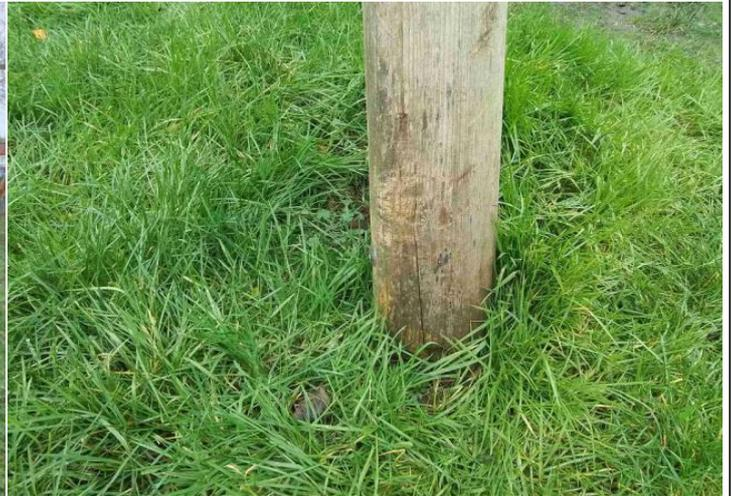
**Finding:** The timber has a number of splits/shakes or air cracks and this may affect the stability or allow water ingress which will accelerate the rotting process
